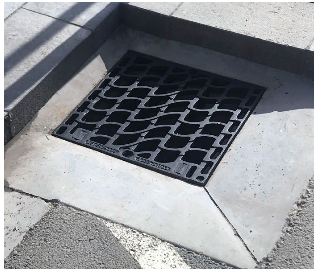
FIG. 1 Hydro 450 x 450mm Grate on standard concrete catchpit
