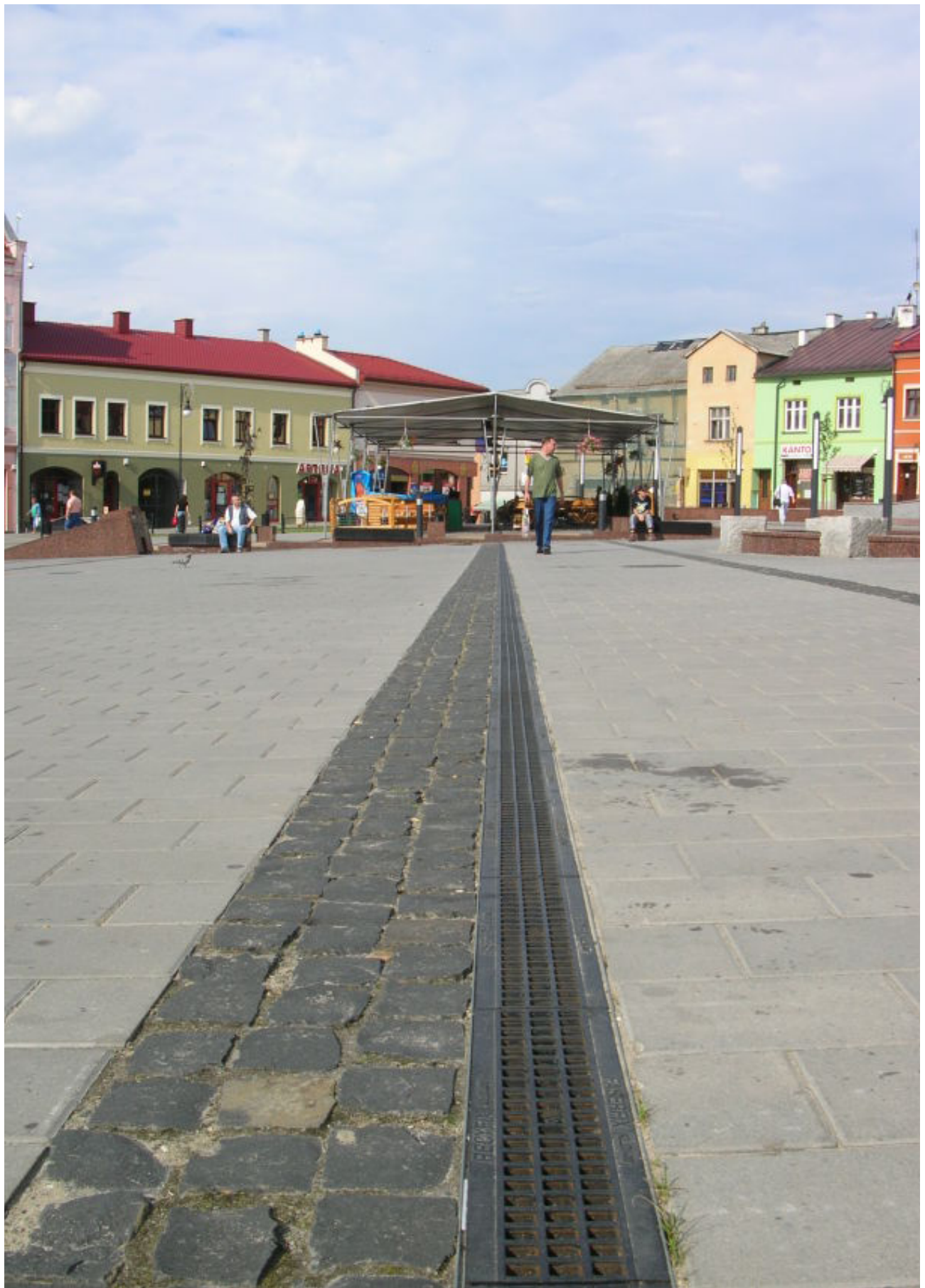
FIG. 36 RECYFIX STANDARD 100 Channel C 250kN with Ductile Iron Mesh 15x25mm Grate
