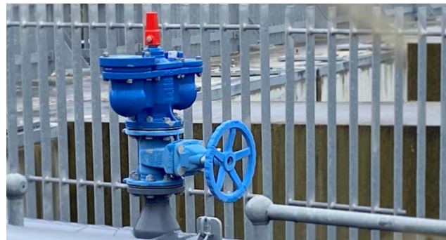
FIG. 1 Combination Air Valve
