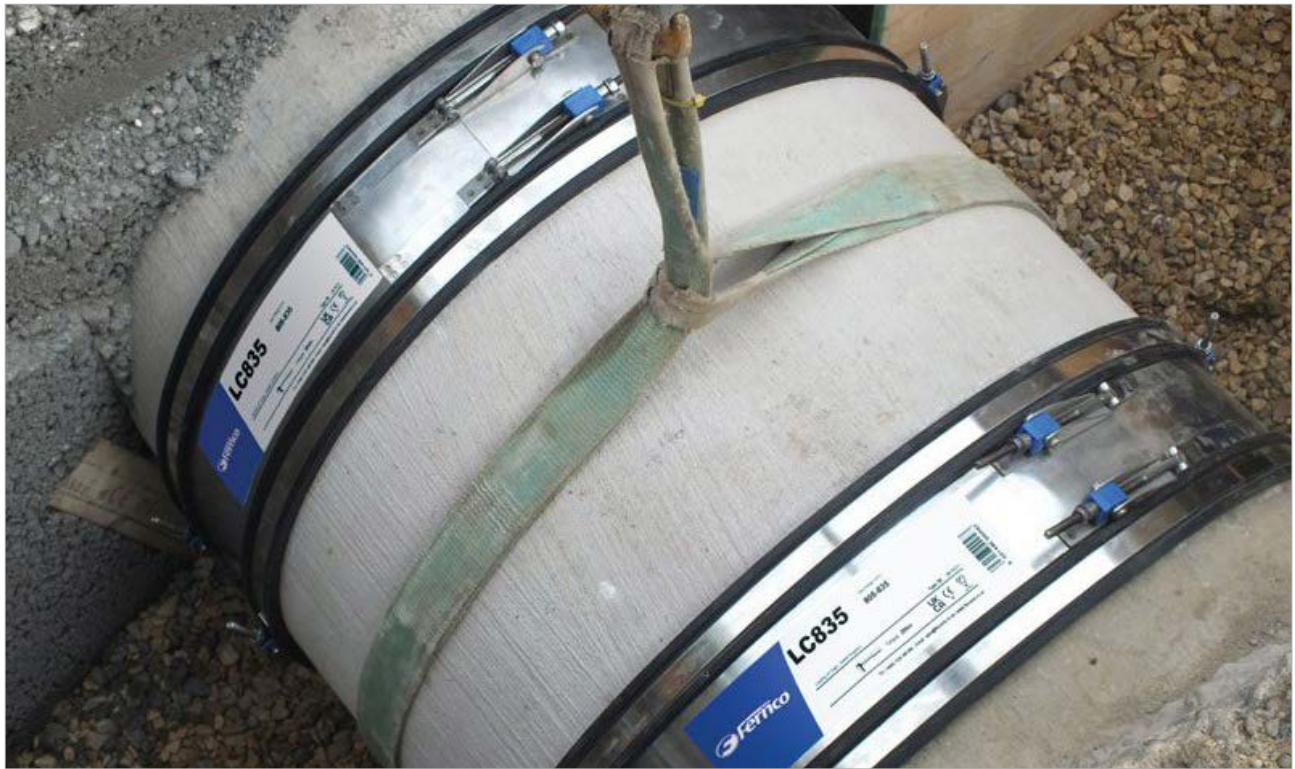
FIG. 2 Fernco Large Coupling insitu installation
