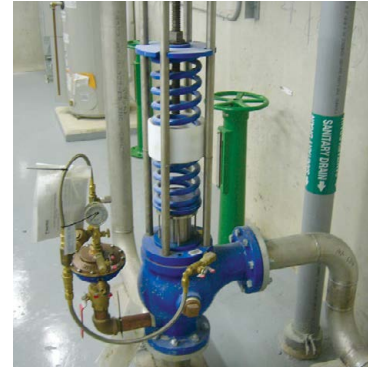
REGION OF YORK (NOBLETON) INSTALLATION ONTARIO, CANADA
